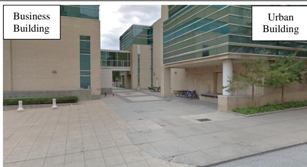
14. Urban Building (UR) – area between UR and BU with picnic tables and bike rack
