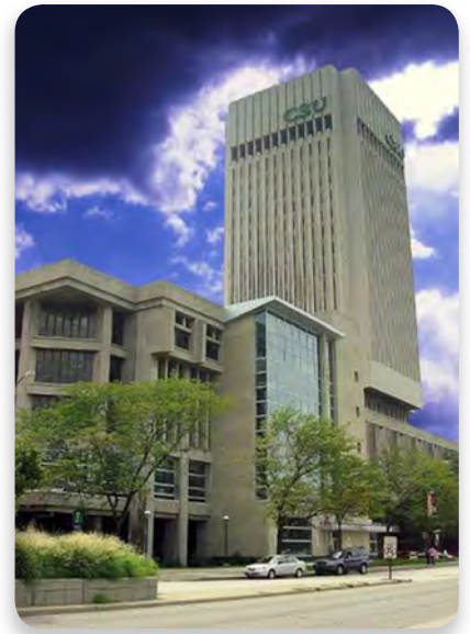
Main Classroom Building
