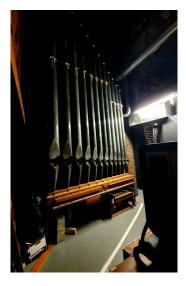
This is a backstage view of some of the pipes for the Severance Hall Norton Memorial Organ. The organ has 6,025 pipes, made of materials such as lead and tin alloy, zinc, and wood and ranging in length from 7 inches to 32 feet.
