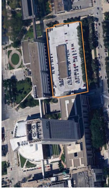
Figure 3.55: Existing Central Garage (View from North)
