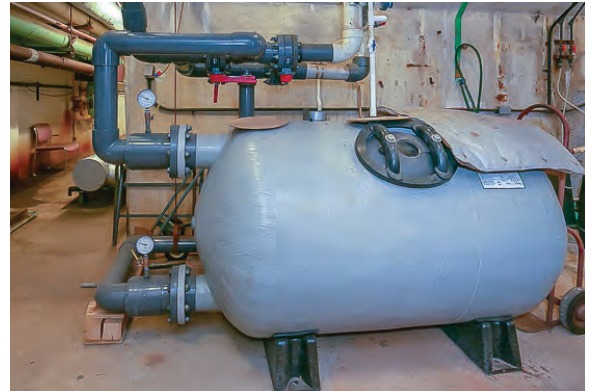
Installation of new small pool sand filter tank and related piping.
