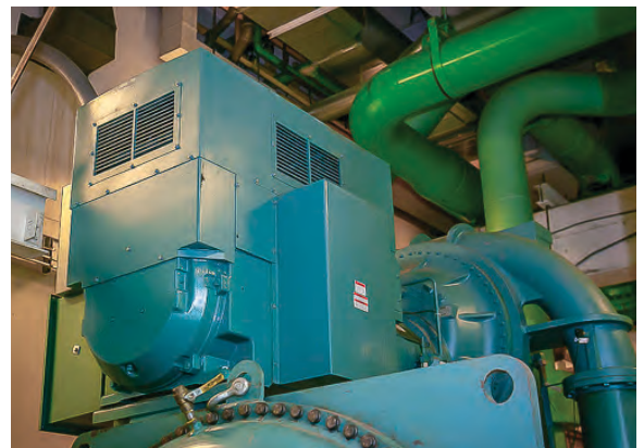
Motor rewind for Chiller #1 Rhodes Tower Chill Water Plant.
