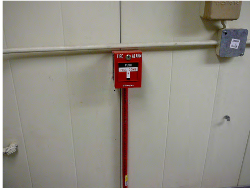
Traditional fire alarm system pull
