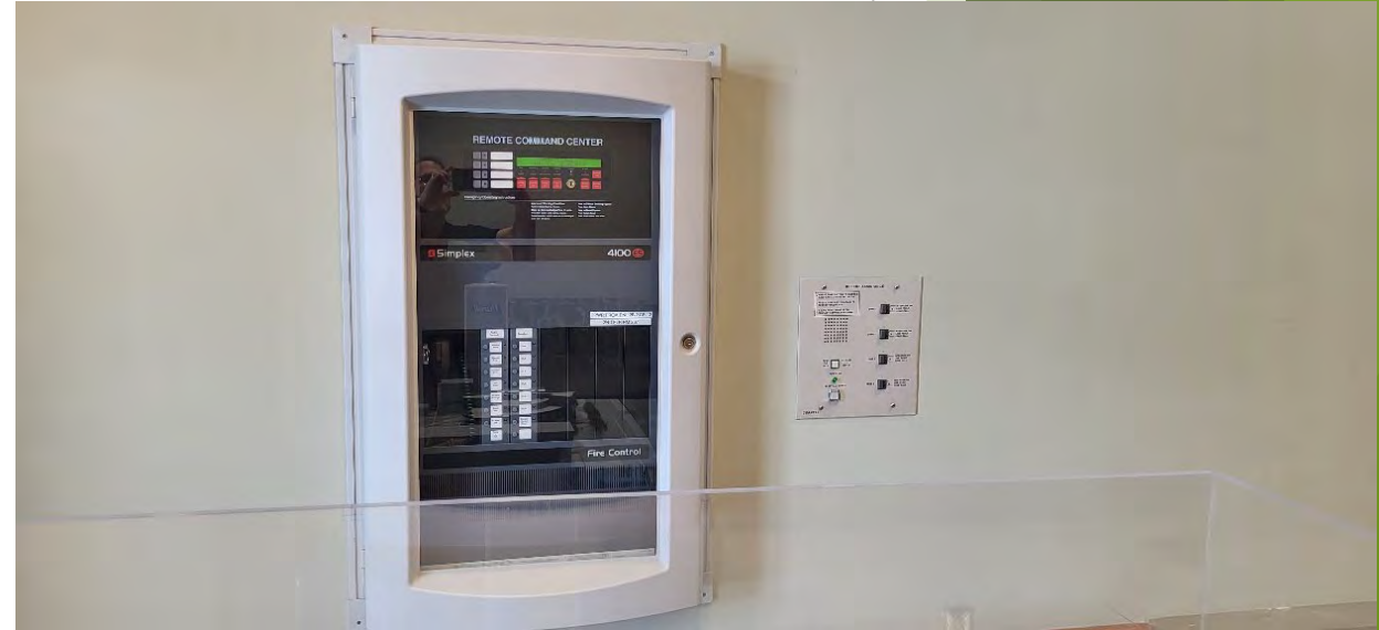
Remote Fire Alarm Panel / AORA
