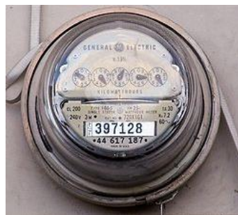
Figure 2 Typical US domestic analog electricity meter, public domain image taken from http://en.wikipedia.org/wiki/Electricity_meter
